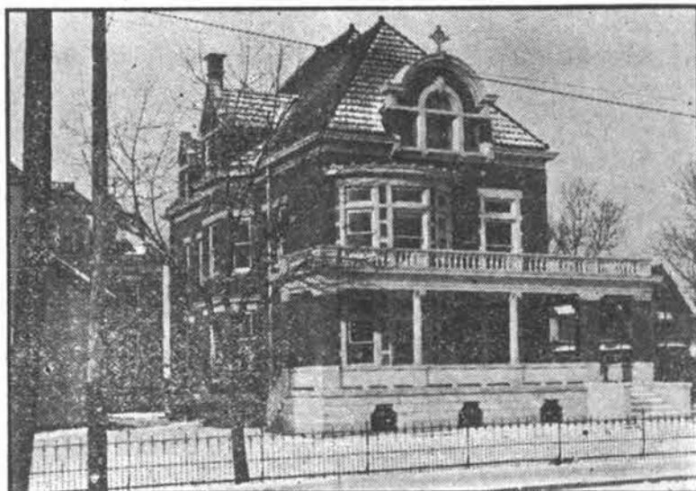
—Photo by Bick. ST. JOSEPH'S CATHOLIC CHURCH RECTORY.
