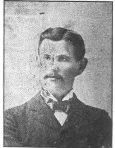
PETER J. LYONS, City Civil Engineer And Superintendent City Water Department.
